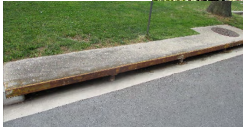
Pavilion drive storm drain
