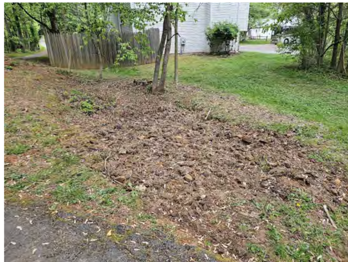
""The Pit"" clean up and fill
